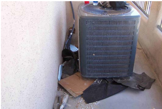
Figure 8.3-9. Remaining debris on north deck. A small amount of water entered into the Crystal Beach SCIP house because there was so much debris on the decks, the drains plugged up, and water entered below the door.
