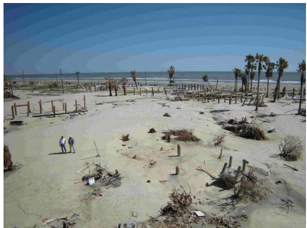
Figure 8.3-8. View looking south towards Ocean, from second floor porch after Hurricane Ike. Four rows of houses were destroyed in front of house 10/18/09 (101809 3720)_
